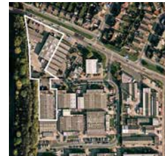
Power Towers's site in Leicester, UK.
